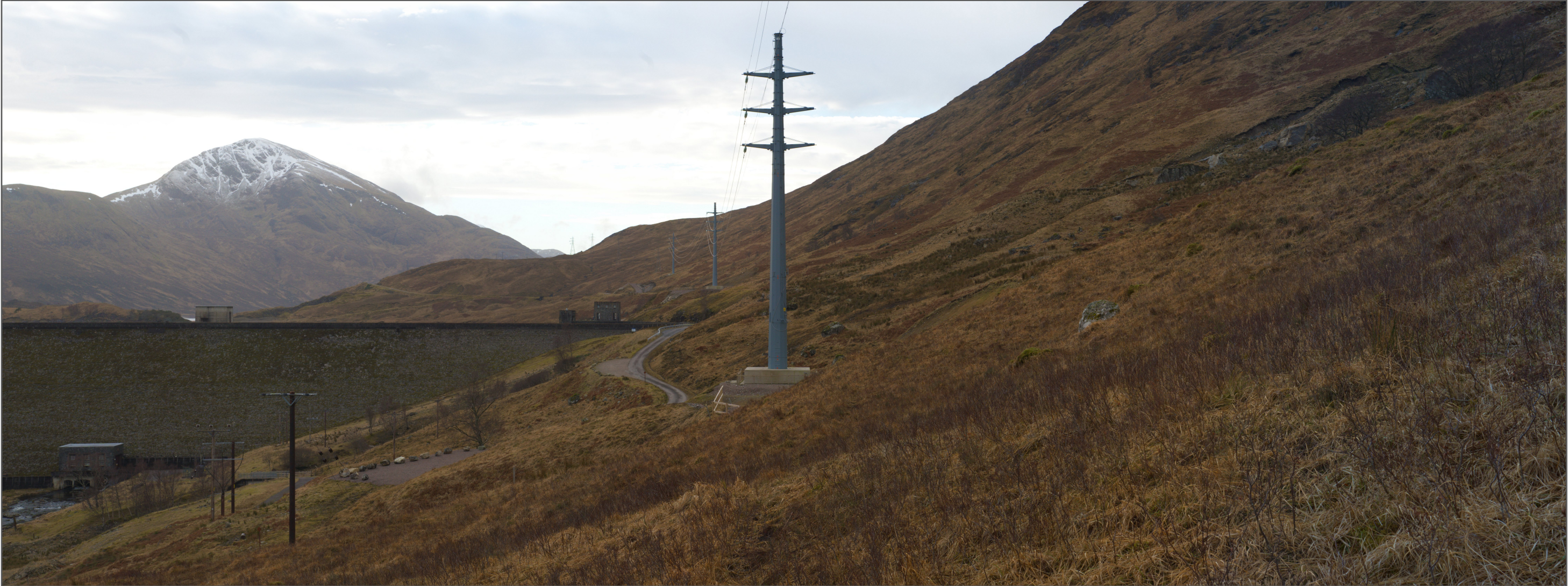
Quoich Repair - TOWER TYPE - NeSTS 132kV DC
