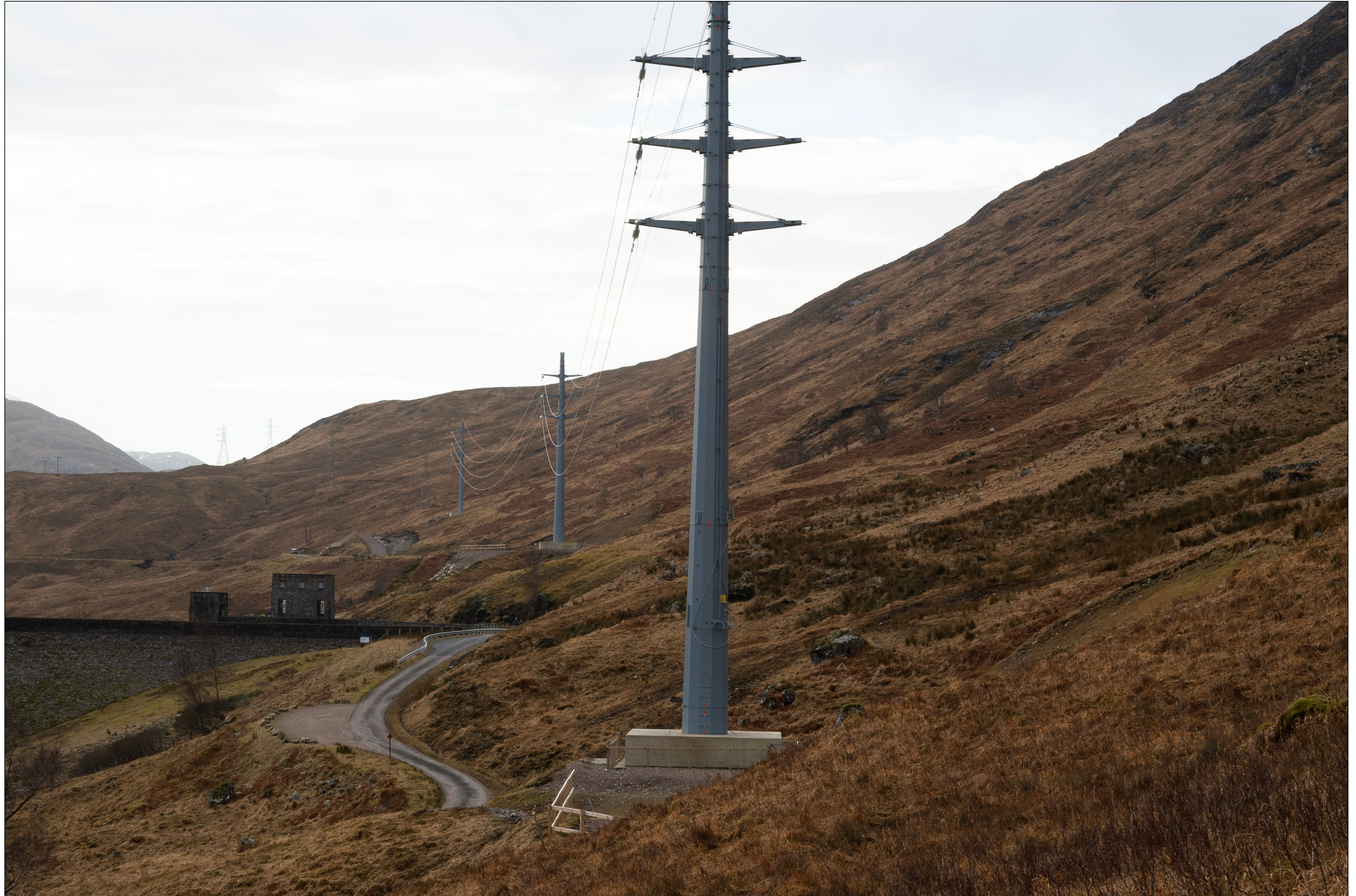
Quoich Repair - TOWER TYPE - NeSTS 132kV DC
