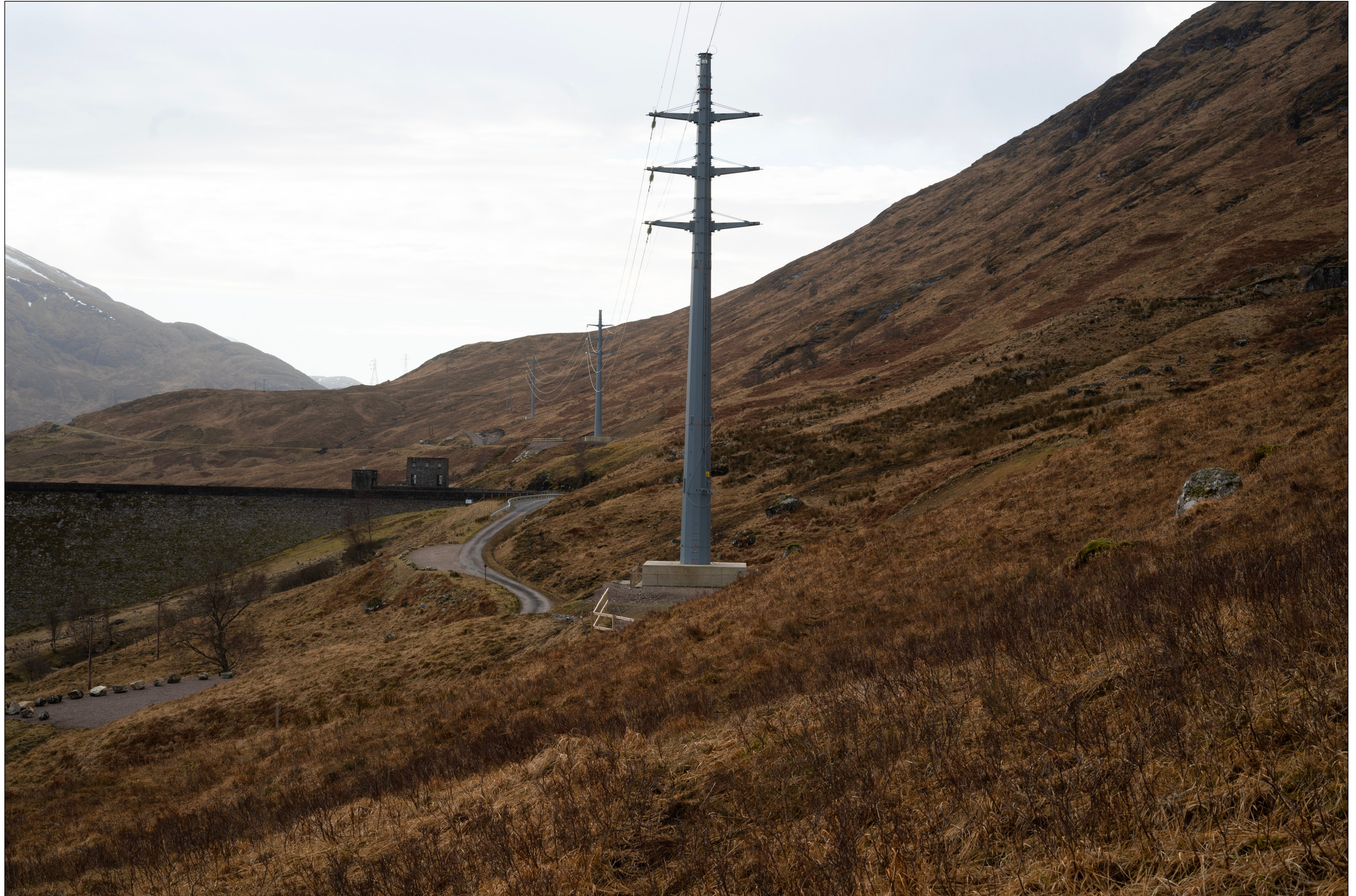
Quoich Repair - TOWER TYPE - NeSTS 132kV DC
