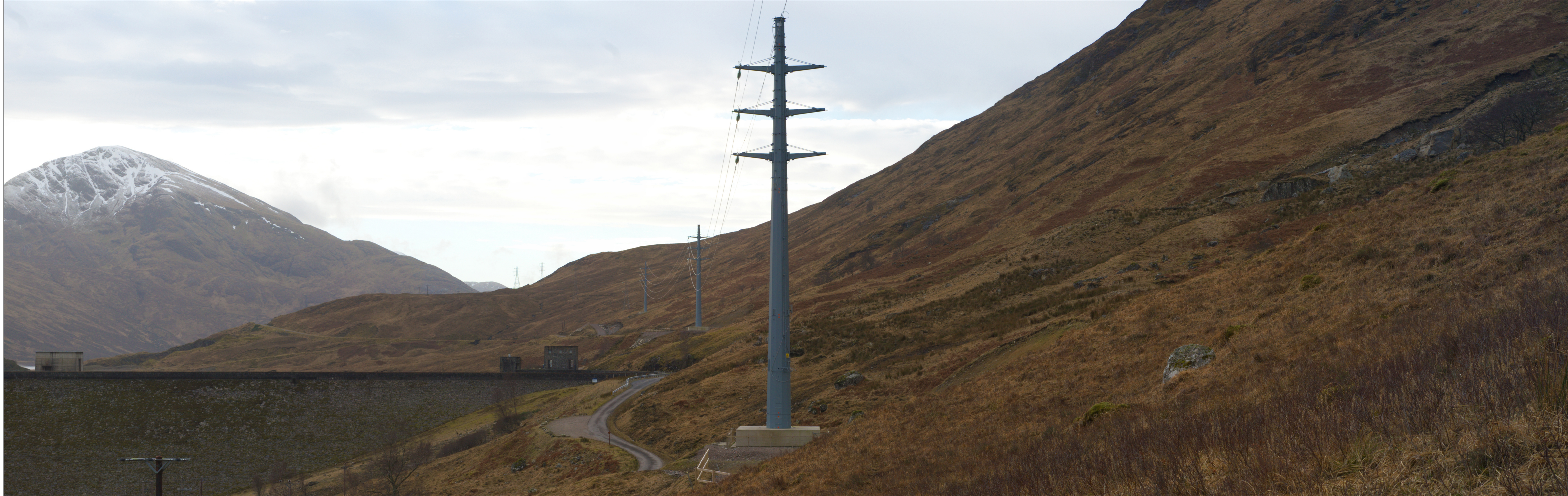
Quoich Repair - TOWER TYPE - NeSTS 132kV DC
