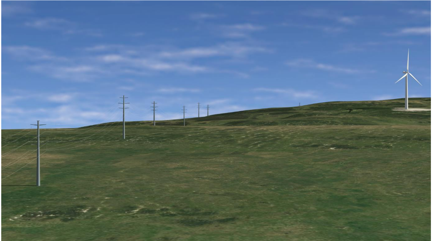
Figure 2: Visualisation of a NeSTS 132kV Double Circuit Medium Duty Overhead line
